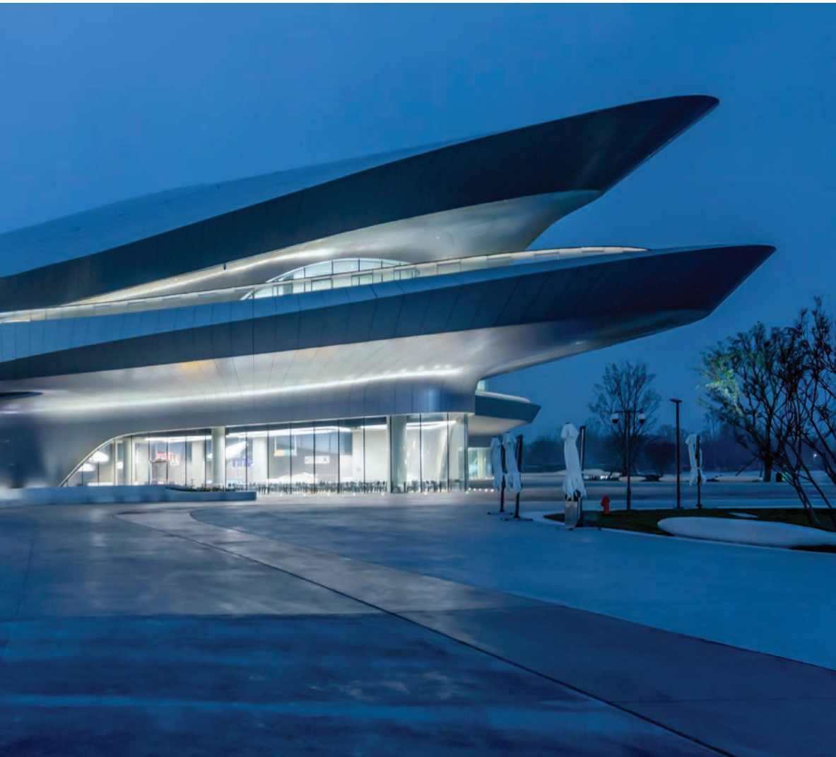
Illuminated glass handrails provide wayfinding and emphasize architecture.
