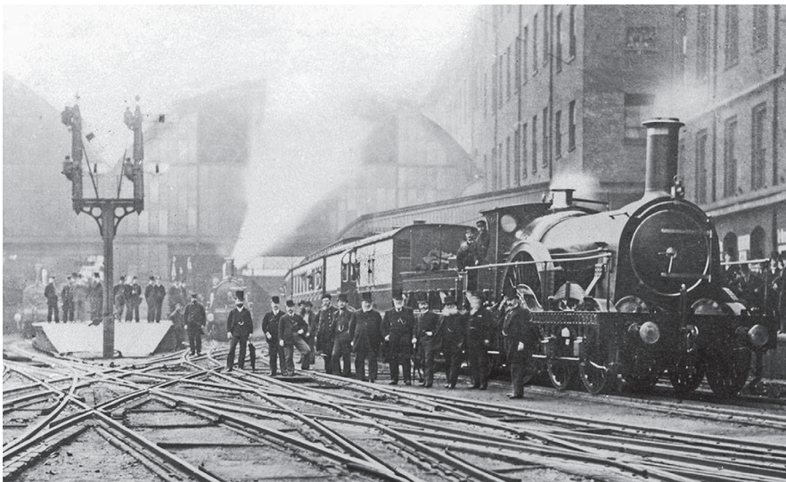
On April 1, 1865, semaphore signals (left) were introduced at Paddington Station in London.
