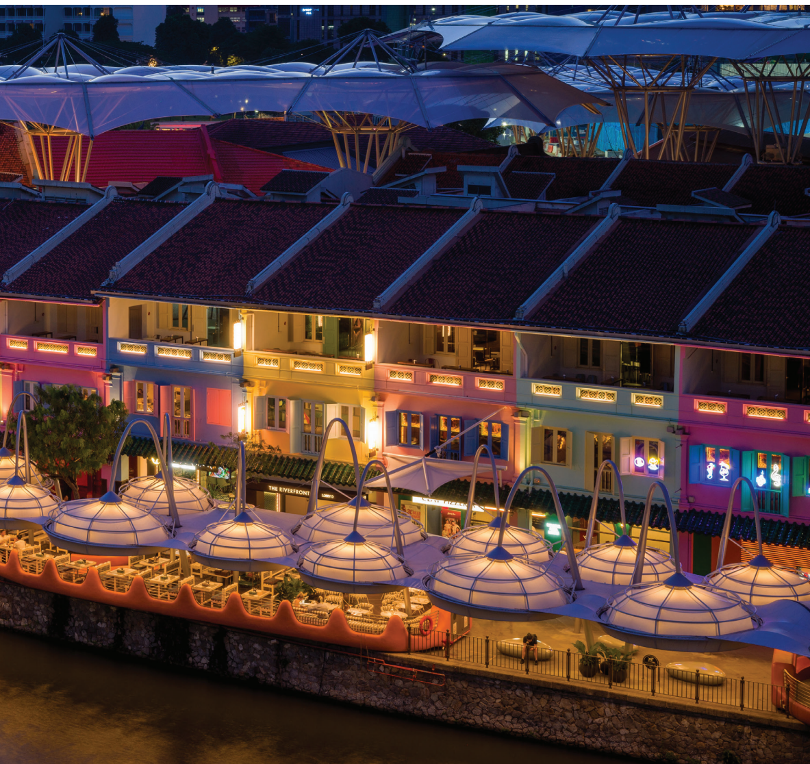
Fabric Bluebell-shaped structures above alfresco dining feature retrofitted warm-white luminaires.
