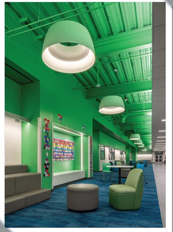
^^ A cozy seating niche exemplifies the multi-layered, flexible lighting scheme , including individually controllable fixtures, glare-free pendants, adjustable wallwashers, and recessed linear luminaires.
